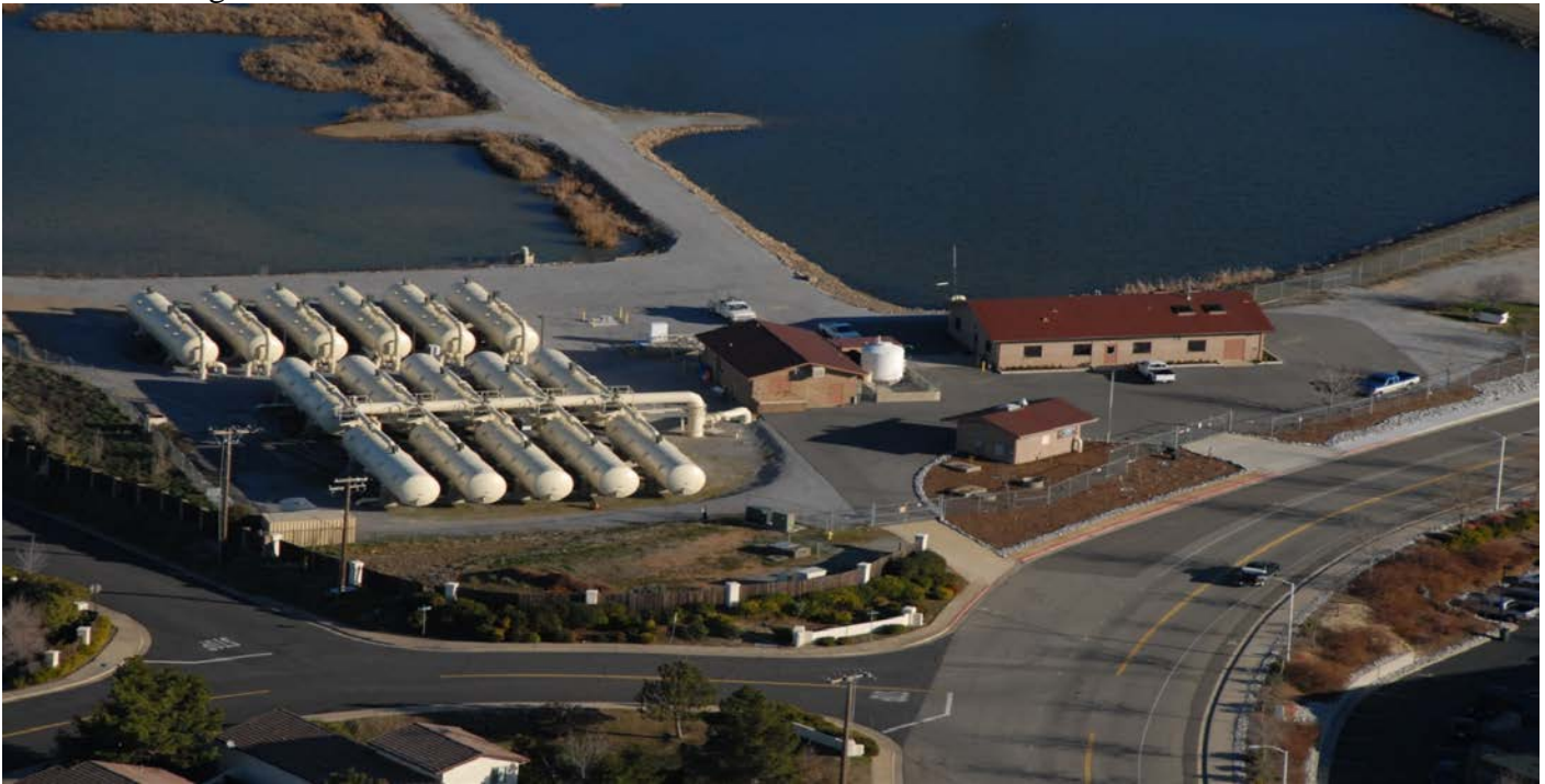
BVWD Water Treatment Plant (60 MGD Capacity)
