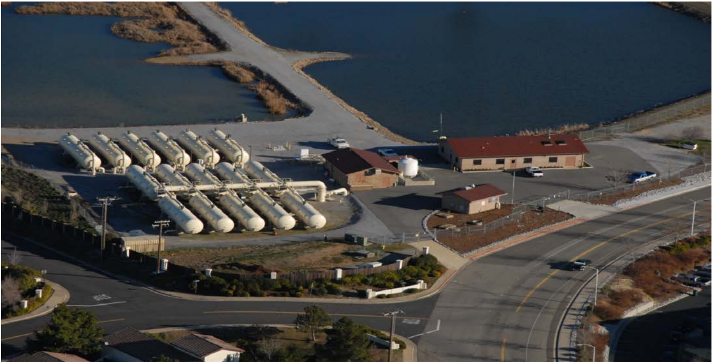
BVWD Water Treatment Plant (60 MGD Capacity)
